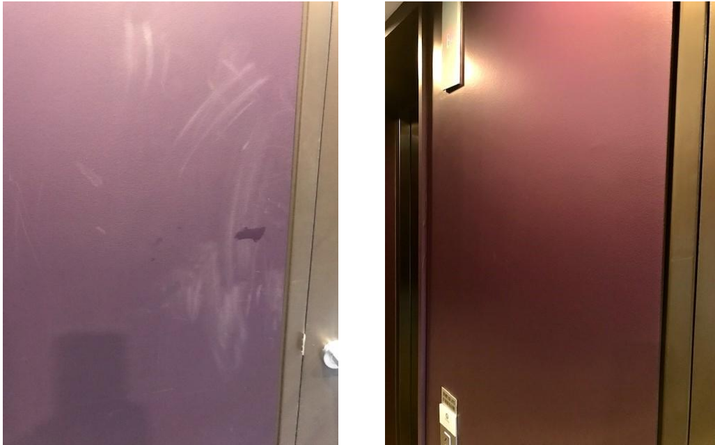
Left: This door shows typical marring. Right: Same door, repainted with Porter's Aqua Satin, and back in use.
